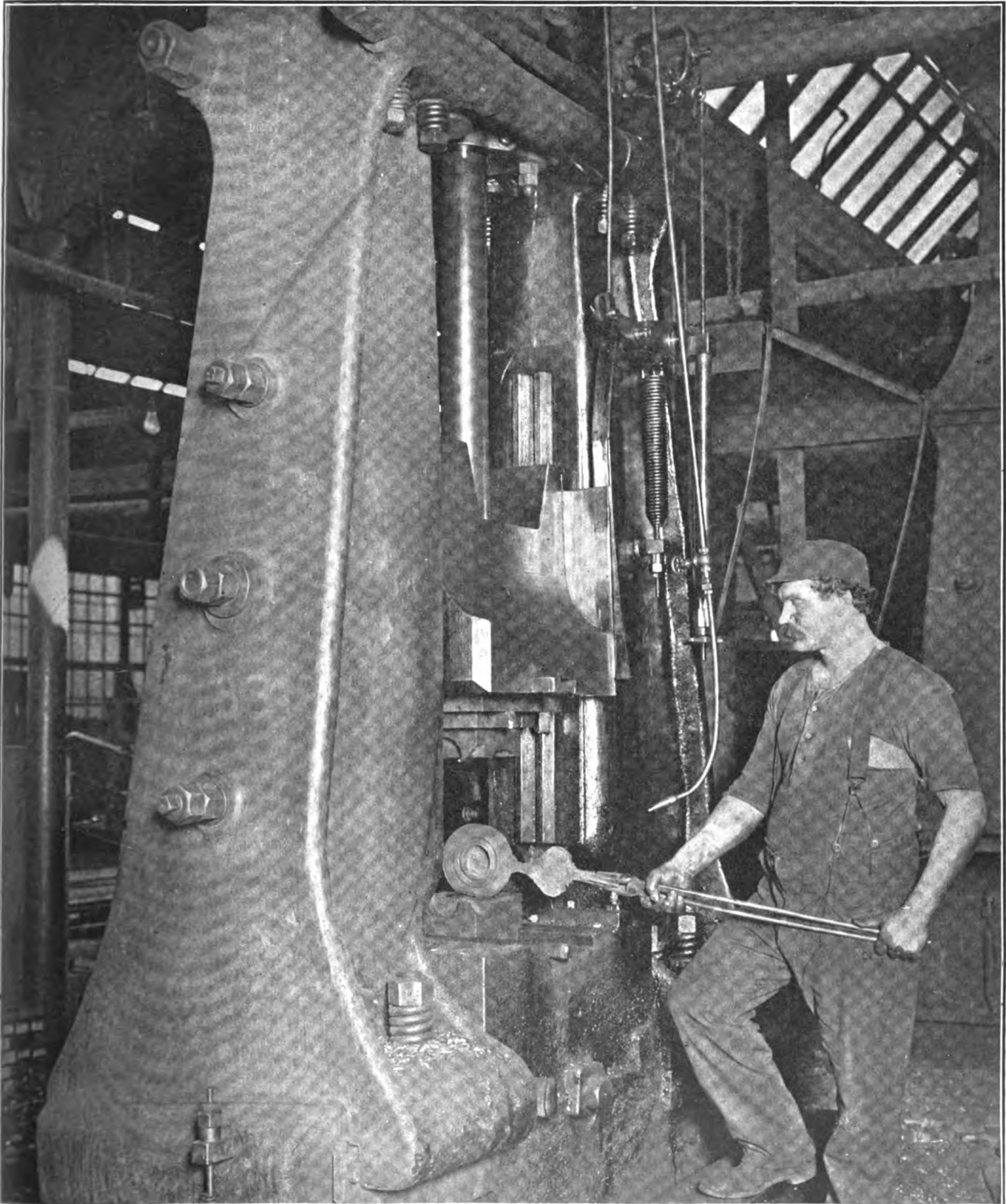
TO AVOID USING INFERIOR CASTINGS ENORMOUS HAMMERS ARE NECESSARY—SCENE AT RAMBLER PLANT
